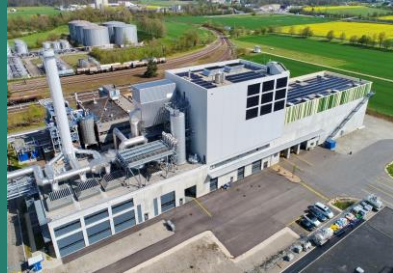
Sisseln biomass plant
